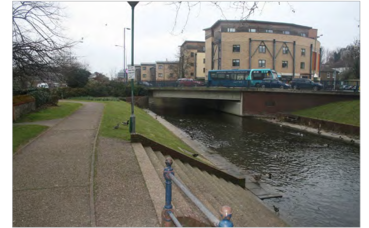
6. Space to the rear of Orchard is framed by backs of buildings, disjointed surfaces, service yards and has poor legibility.
