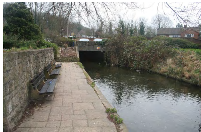
Poor quality and segregated river frontage - Bridge House Gardens
